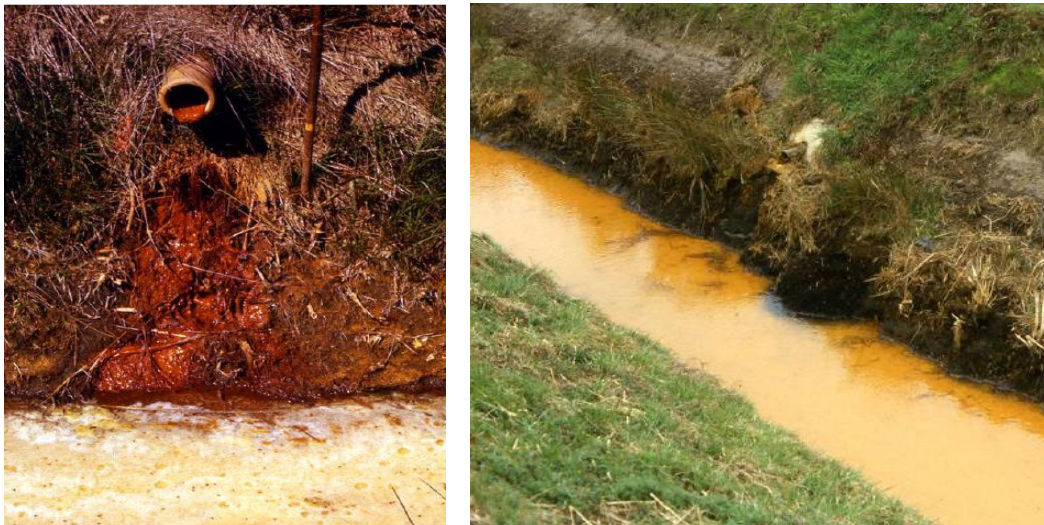
Ochre in Fenland drains and watercourses © Rodney Burton
